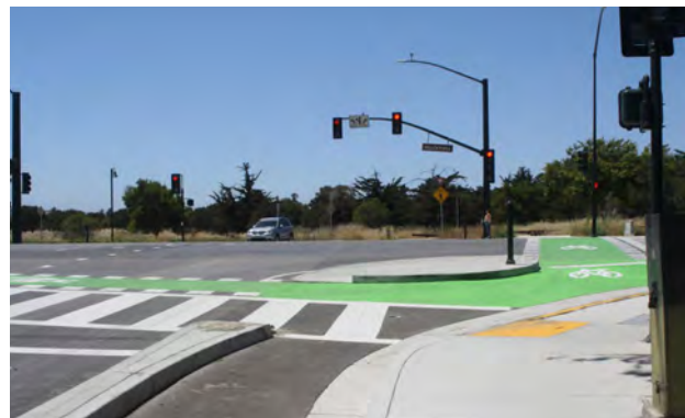
Protected intersection for bike and pedestrian crossings
