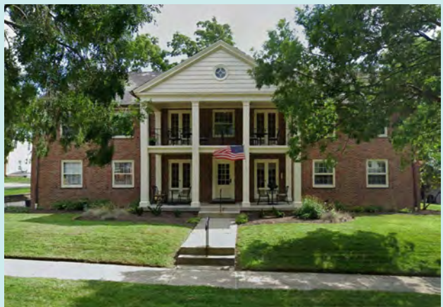
Existing four-family home
