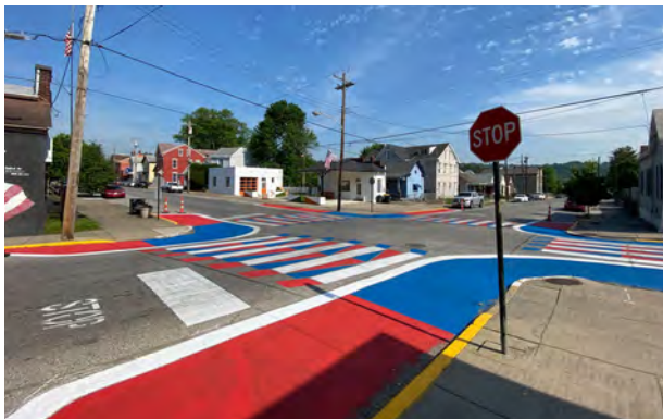
Quick-build or temporary curb extensions
