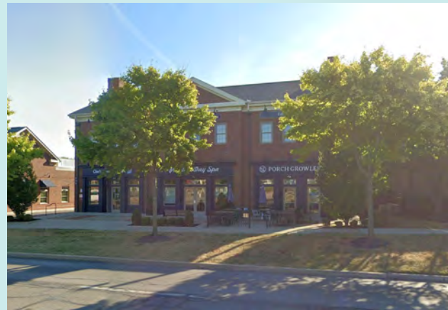
2-story commercial building near North St and High St
