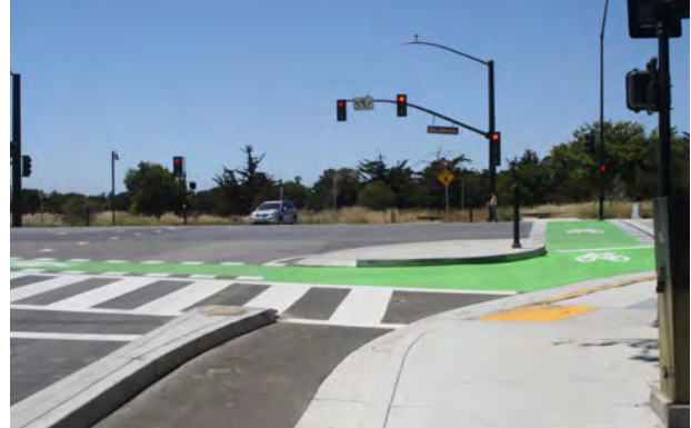
Protected intersection for safer bike and pedestrian crossings
