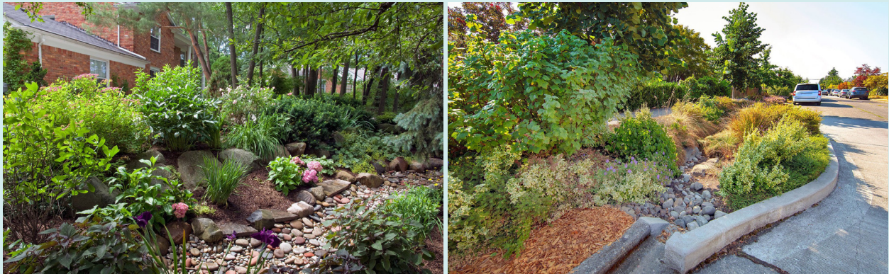
Low-impact stormwater management techniques like rain gardens (left) and bioswales (right)
