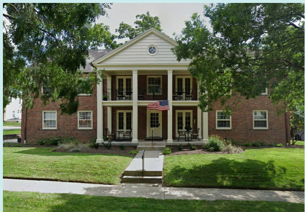
Existing four-family home
