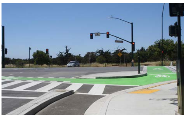
Protected intersection for bike and pedestrian crossings
