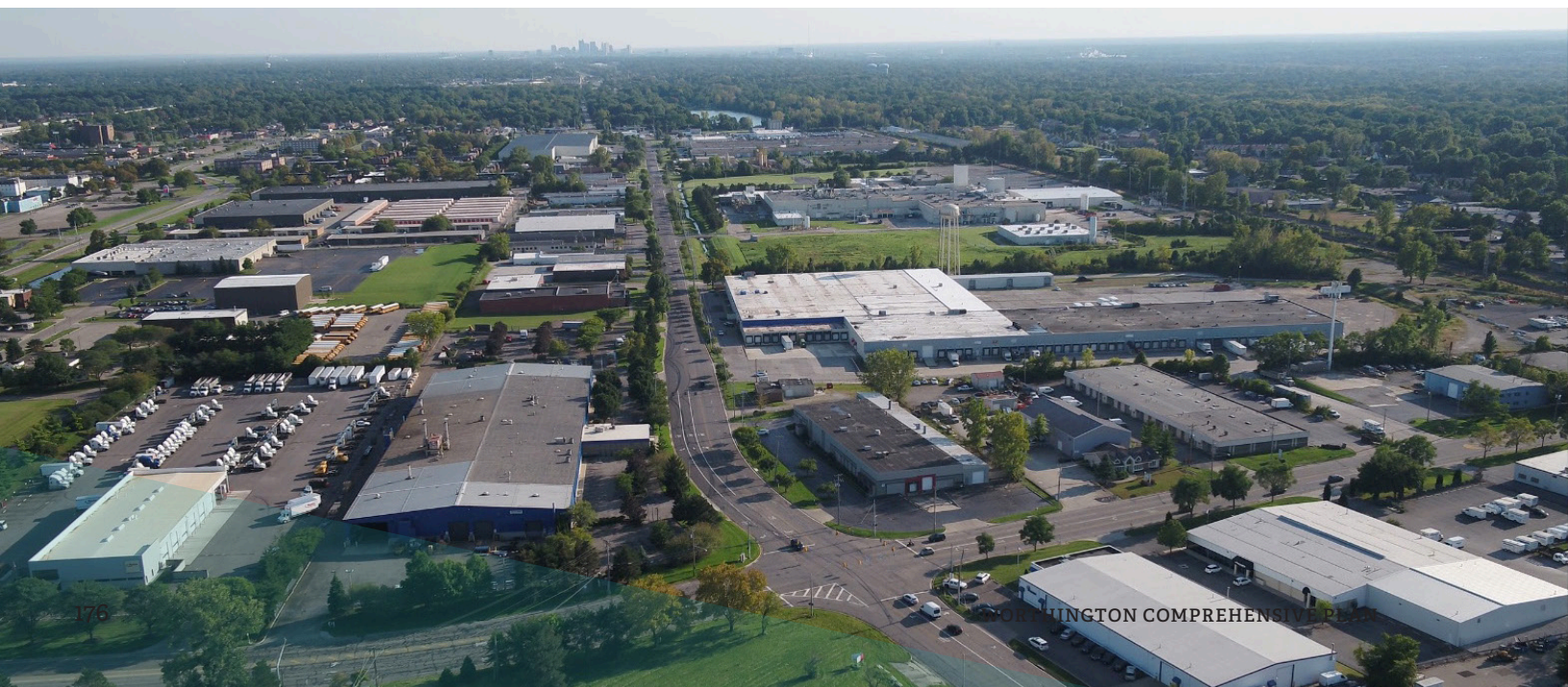
Aerial of Huntley Rd looking south towards Columbus
