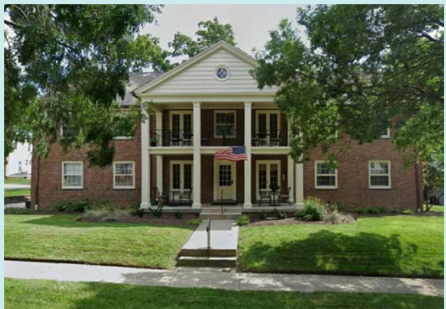
Existing four-family home
