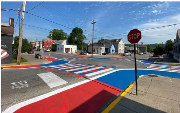
Quick-build or temporary curb extensions
