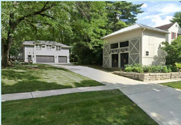
Existing carriage house
