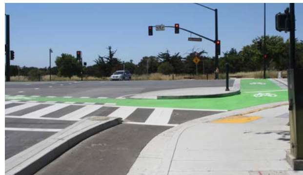
Protected intersection for safer bike and pedestrian crossings
