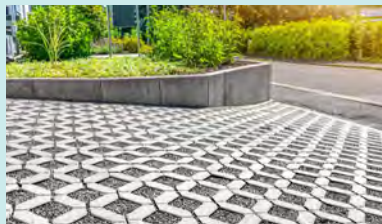
Permeable pavement: surfaces that allow water to infiltrate rather than run off, reducing peak flows and downstream flooding risk
