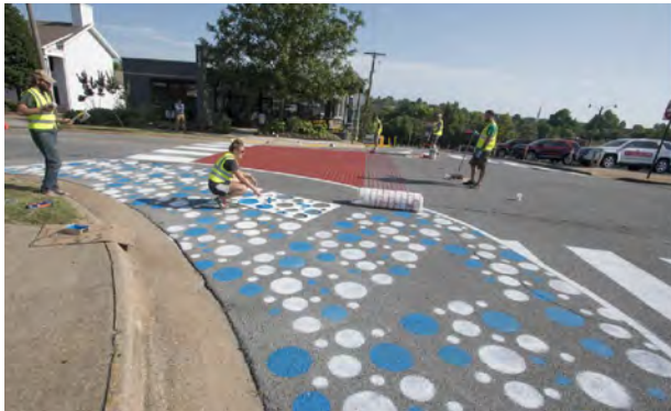
Temporary curb extensions at an intersection using paint (left), and same intersection after permanent infrastructure was installed (right)
