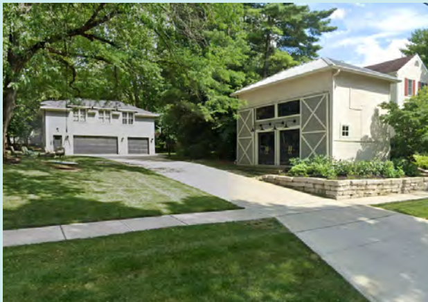
Existing carriage house
