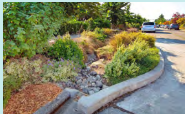
Bioswales: vegetated channels that slow and clean stormwater along roadways and corridors
