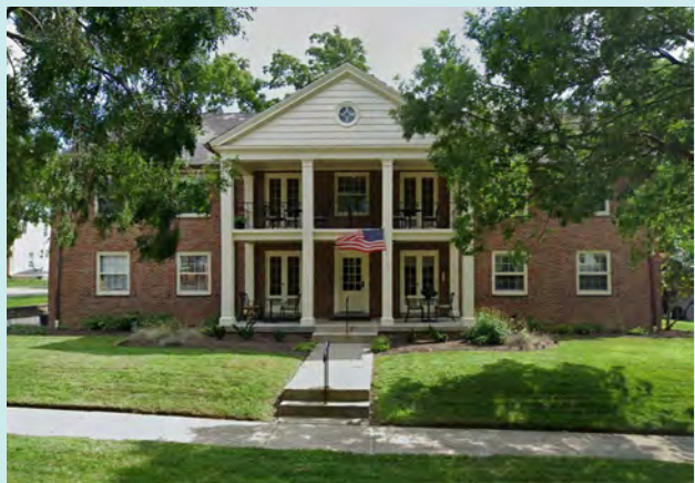
Existing four-family home
