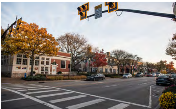
High Street crossing south of the Village Green
