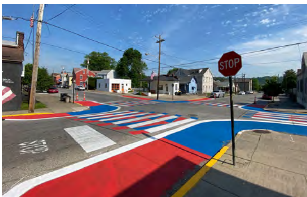
Quick-build or temporary curb extensions
